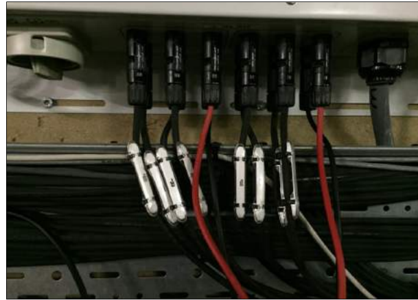
Figure 16 : Connection to available inputs
